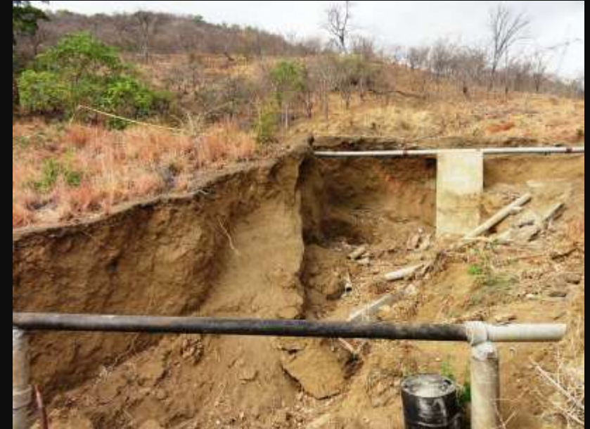
"Destroyed water and sewer pipes by elephants in Kariba" by Sustainable sanitation is licensed under CC BY 2.0 .
